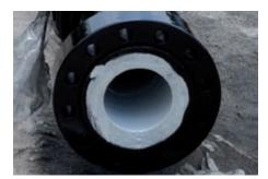
First of all, the pipelines were grit blasted according to standard SSPC-SP10 by special pipe interior sandblasting equipment with rotating head.
