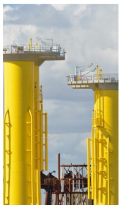
Rotor frames, rotor blades and towers of offshore wind generators have to withstand extreme weather conditions. The constantly moist and salt-laden air combined with intensive UV radiation is highly corrosive. Tremendous wind speeds and rainstorms with an impact of hammer strokes induce heavy wear and abrasion effects. Due to tides and waves foundation piles are exposed to high corrosion risk and severe mechanical friction.
