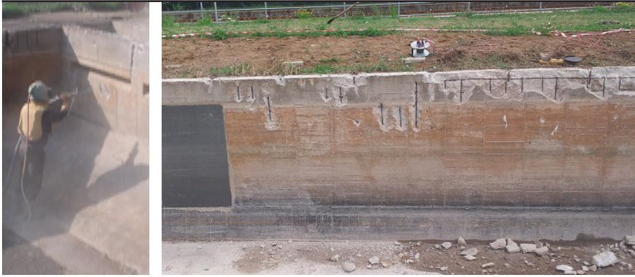
Grit blasted area, loose concrete was removed
