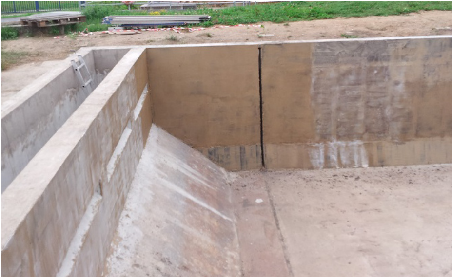
Rebuilt top edge, application of the primer
