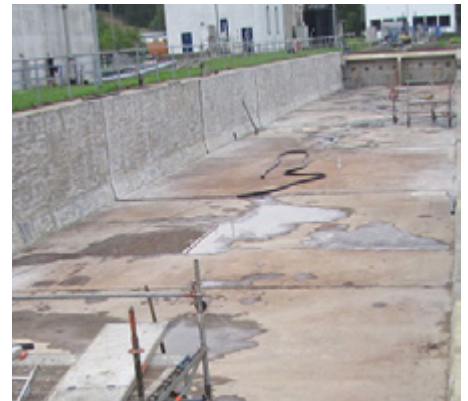
Grinded wall area
