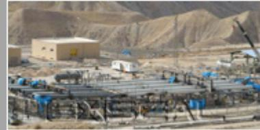
During the extraction, natural gas is very humid and therefore highly corrosive. Due to the high pressure (in this case 250 bar) and absorbed debris, intensified abrasion occurs on the internal walls of the whole pipeline system. Moreover, the temperature of approximately 60°C (ambient temperature) and the aggressiveness of the hydrogen sulfide demand an absolute high quality and resistant coating system for the internal lining of the gas conveyor plant.
