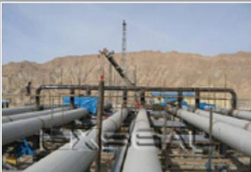
For "Tange Bijar" project a multi-pipe slug catcher (finger-type) is assembled. The conveying tube is extended in parallel pipelines, each with a diameter of 56 inch (1,42 m) and a length of 80 m. In these "fingers" the volume expands and the gas reduces velocity. Due to the lightly falling gradient of the pipes, debris and humidity settle in special catchment tanks and can be removed separately.
