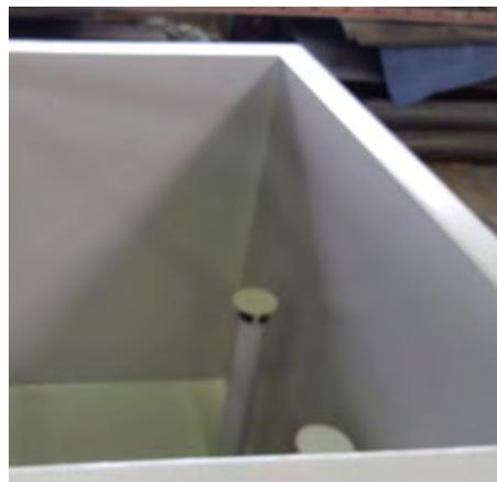
In Germany, the Waste Water Ordinance forbids the disposal of toxic substances into the sewage system. Service water from the parking garage, which is contaminated with oil residues and chemical detergents, must not get into effluents without filtering. Thus, a suitable collecting container and 2 big activated carbon filters are applied for the cleaning of the process water in the car park.
