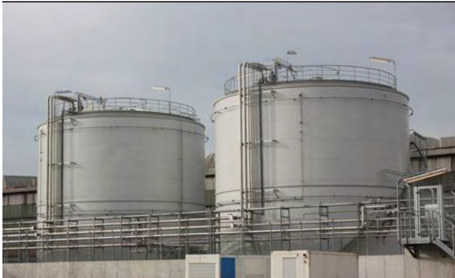
Exterior view of the tanks after 5 years! The coating is still intact. No weathering effects or corrosion damages occurred on the exterior walls of the tanks.
