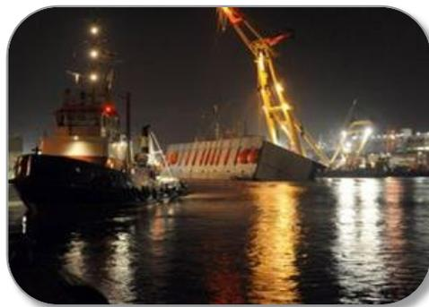
For coating the huge lock gates our versatile product **Ceramic-Polymer SF/LF** was selected. In the high flow rate area there is an intensified occurrence of abrasion, also presence of accelerate risk of corrosion due to the increased oxygen content of the lock water. High class corrosion protection and extreme abrasion resistance of **Ceramic-Polymer SF/LF** guarantee the long life-cycle of the gates.
