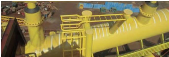
There is a high corrosion risk within the splash zone of offshore constructions. For the durable corrosion protection our coating product “Ceramic-Polymer SF/LF-SRB” was applied directly on the steel substrate.
