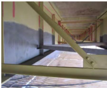
Our coating product Proguard 96 (color „sand yellow“) was applied by airless spraying on the prepared substrate. One layer of 200 µm is adequate to provide an outstanding corrosion protection.
