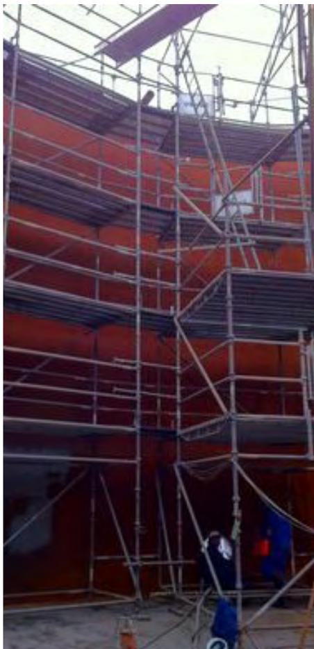
Both open steel tanks had wall and floor surfaces of 1.000 m<sup>2</sup>. After pre-treatment (sandblasting, SA 2 ½) the coating was applied simply by airless spraying methods.
