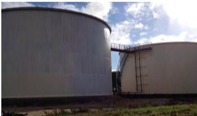
Until further processing, the highly corrosive liquid is intermediately stored in these tanks with a temperature of 60°C. Therefore, high requirements for corrosion protection are placed in this field of application.
