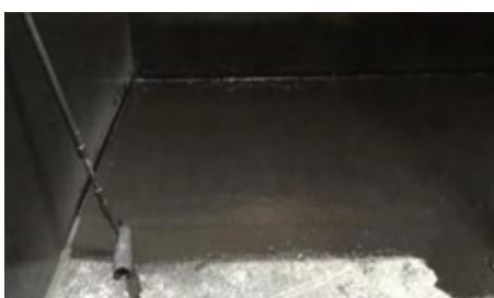
Concrete and steel constructions of digesters, septic tanks, slurry reservoirs, fodder fermenting silos, biogas and composting plants as well as wastewater systems are constantly exposed to high chemical attack by acidic contents of the storage substances. Concrete erosions of 1 to 2 cm and extreme corrosion damages on all steel components are measured per year.
