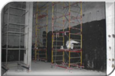
For the Efes brewery in Novosibirsk/Russia the indoor premises for the waste-water treatment facility were coated completely with high quality products of our **Proguard-Series**, to attain a resistance of the concrete against chemical attack. A Ceramic Polymer supervisor observed the preparation of the concrete as well as the application of the coating material and supported the practical use of our products with competent advice.
