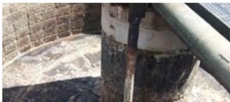
The damaged concrete was removed and the cracks were specifically clamped. Then the complete area was sandblasted and concrete erosions were filled accurately.
