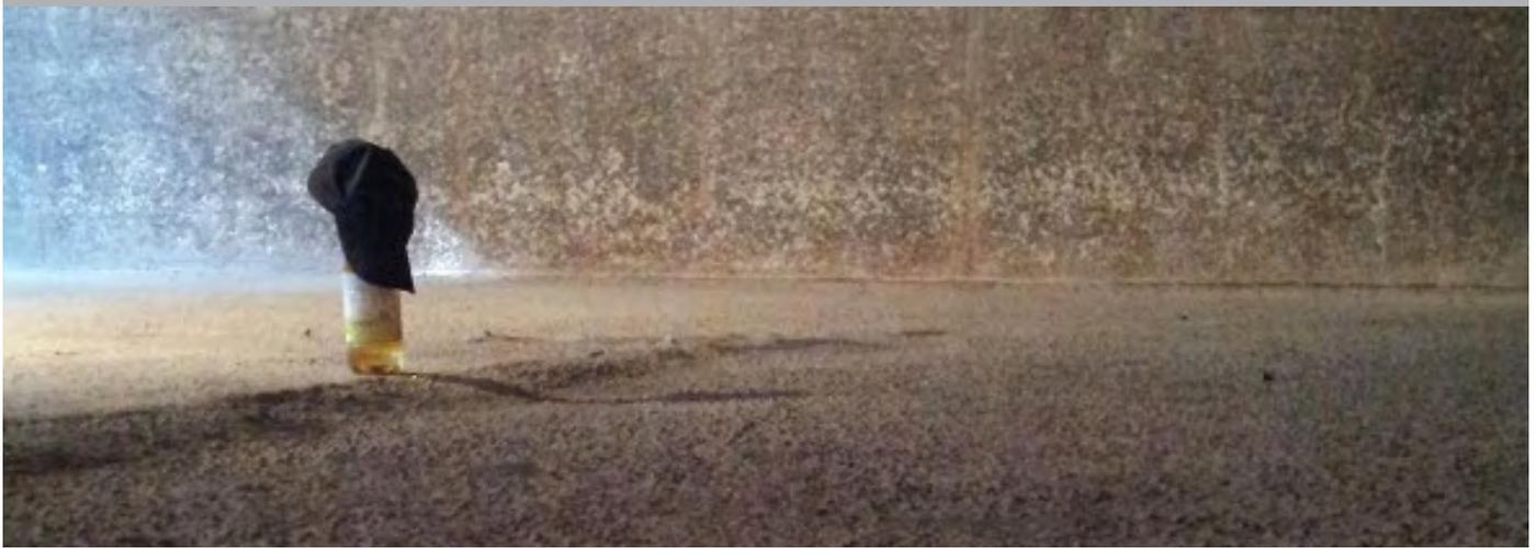
» For applications within the range of wastewater treatment and biogas techniques protective coatings should provide high-grade chemical and abrasion resistances. The concrete substrates in the storage room showed deep erosions caused by the chemical attack of aggressive biogenic waste material. The chamber was renovated with our concrete protection systems to ensure durable operation and value preservation.
