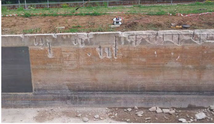
Grit blasted area, loose concrete was removed
