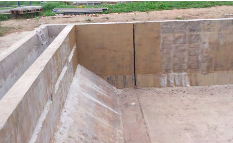
Rebuilt top edge, application of the primer
