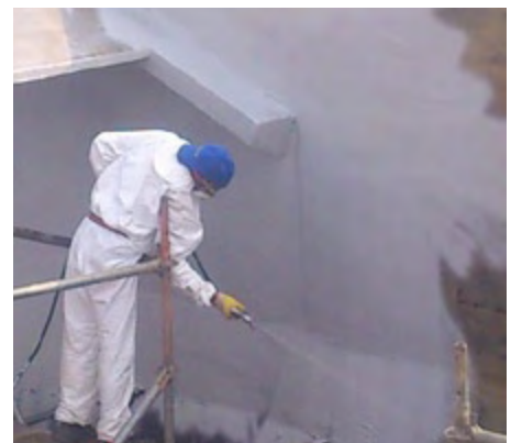
Application of the coating PROGUARD CN 200
