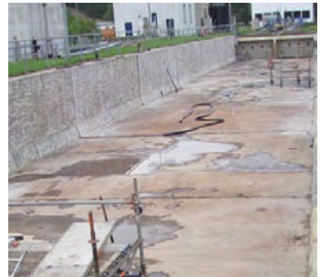
Grinded wall area
