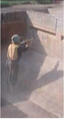
Grit blasted area, loose concrete was removed
