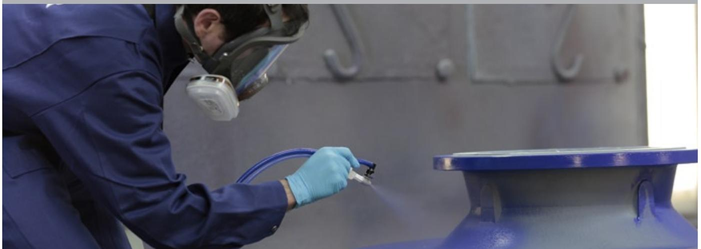
» We now offer efficient cartridge application for some selected products. We decided to implement the advanced Mixpac technology from the company Sulzer to simplify the complex coating application procedure significantly. An optimum solution for repairs, small projects or areas which are difficult to access!
