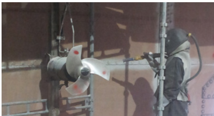
Firstly, the area was sandblasted.
