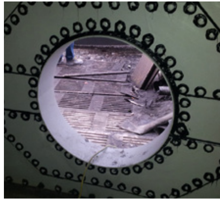
Extra, flexible sealing of rivets, welds and abutting edges.
