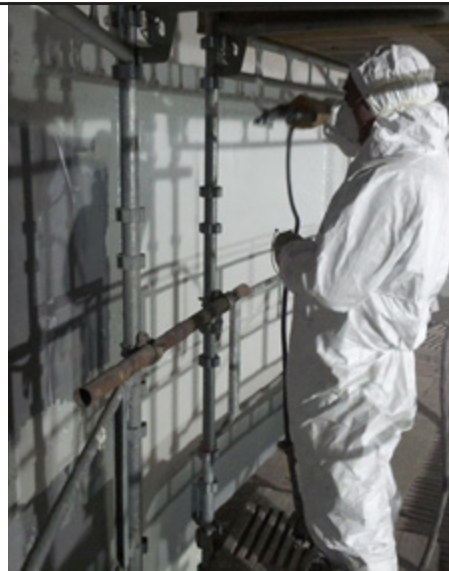
Application of the coating system PROGUARD CN 200 by airless spraying.
