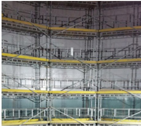
First section completed – the upper area is coated.
