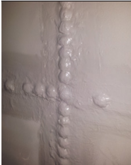
Pre-coating of welds and rivets with PROGUARD CN 200.
