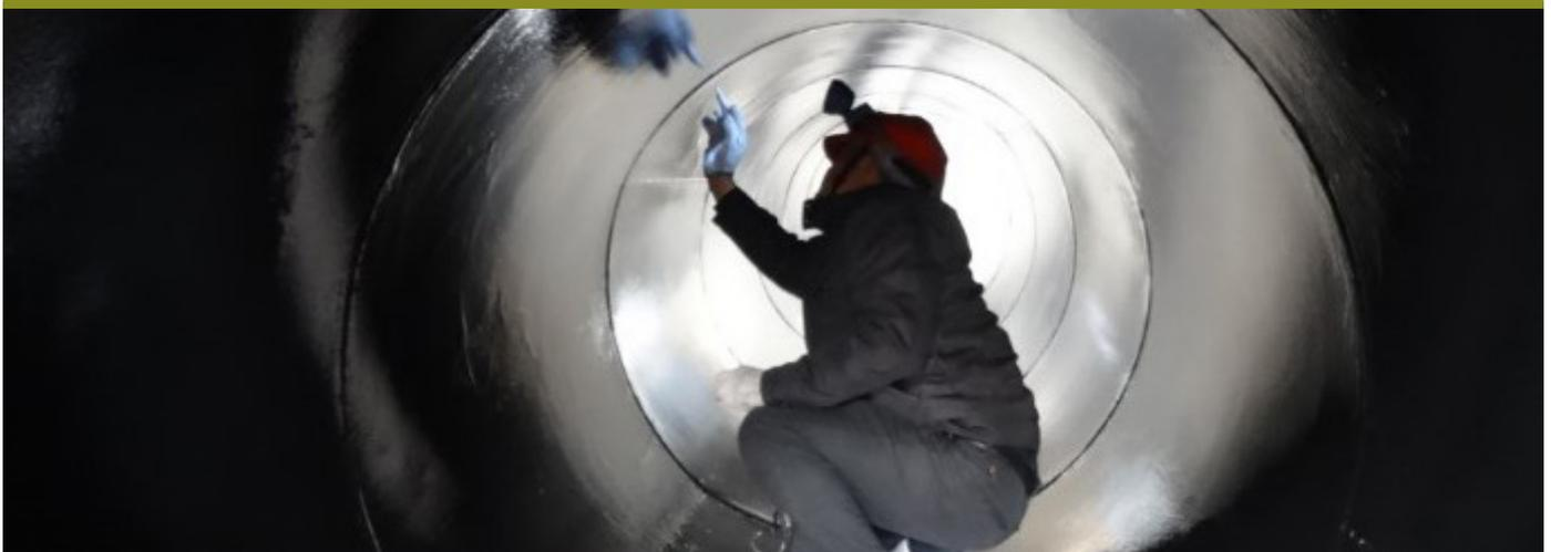
China: The chimney of a waste incineration plant was protected with our chemically resistant premium coatings against aggressive influences of the cleaned flue gas. Before the application was conducted, sample plates of PROGUARD CN-OC and PROGUARD CN-1M were subjected to a long-term-test and placed into the inner chimney. No corrosion and peeling occurred on the coated plates; therefore, our coating systems were selected for this demanding project.
