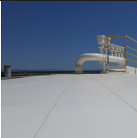
Roof with applied coating and top coat.
