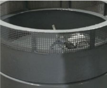
Before the protective coating was applied the surface was again sandblasted. The repaired areas were roughened by sweeping. The application of **CERAMIC-POLYMER STP-EP-HV** was conducted in 2 steps: pre-coating of edges, ventilation screens and blades was passed with brush or roller to increase the total layer thickness in these sensible zones. Following, the coating was applied by airless spraying with a thickness of 350 µm. The curing time was also 20 hours at a room temperature of 20 °C.
